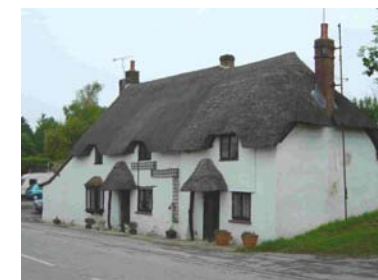
Fig 52. Nos 67 & 69 Main Rd
