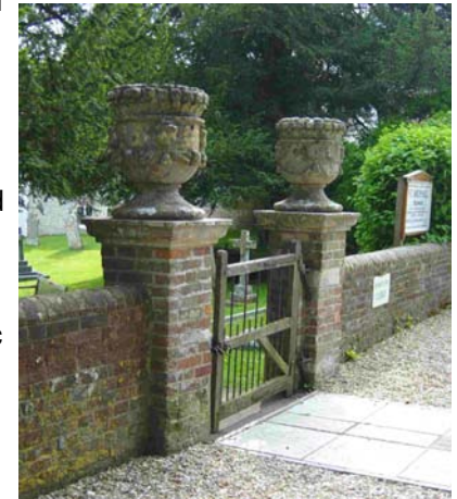
Fig 41. Gated entrance to parish church
