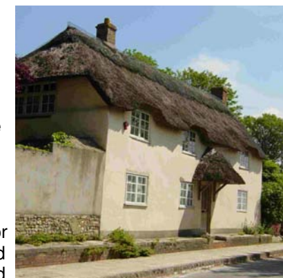
Fig 58. No 25 Dorchester Rd with thatched roof and door canopy and casement windows
